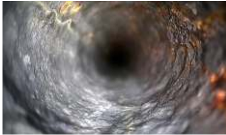
Real life problem 2 Corrosion of Piping
